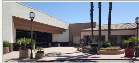
P-19 storefront / signage condition
