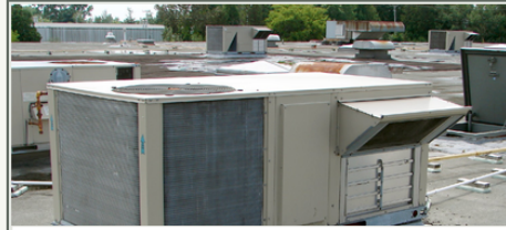
P-08 rooftop HVAC condition
