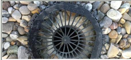
P-03 roof drain / ponding check
